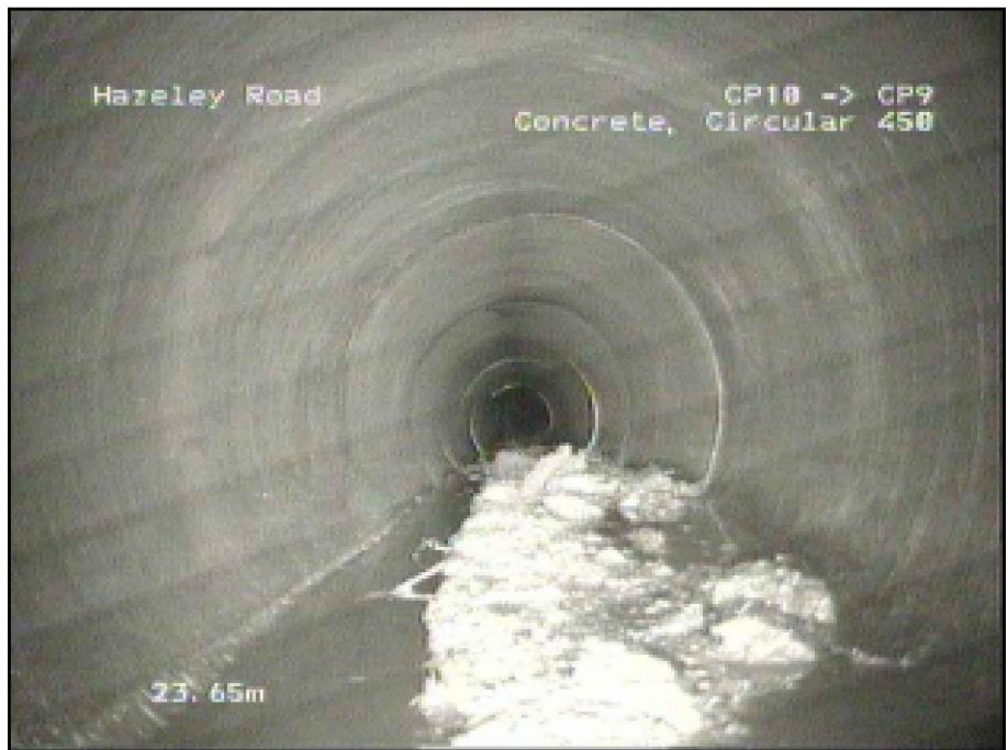
Large amount of settlement in sewer
