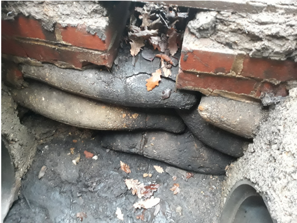
Figure 3.7 – Concrete Sandbag Manhole
