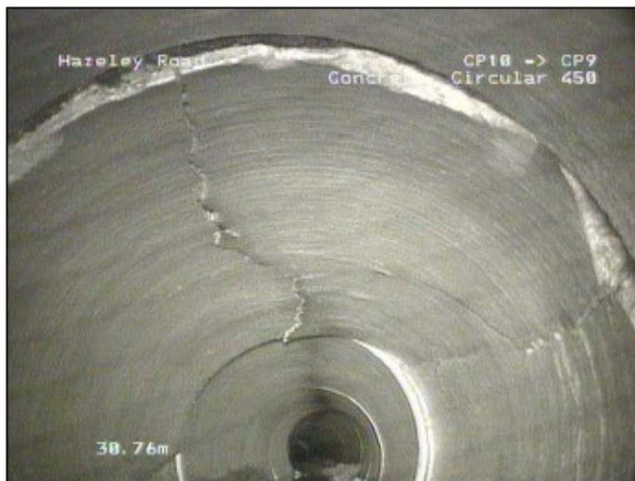
Figure 3.4 – Longitudinal cracking
