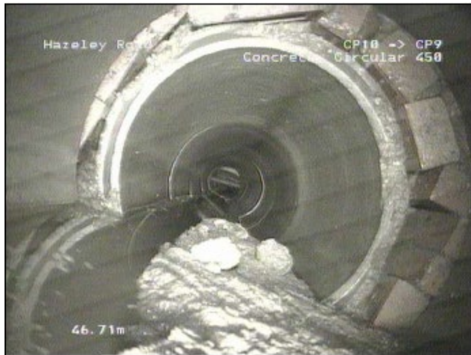
Figure 3.8 – Sewer Settlement
