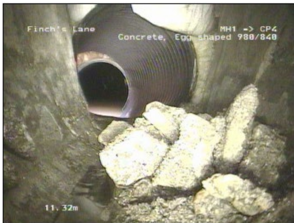
Figure 3.9 – Sewer Settlement
