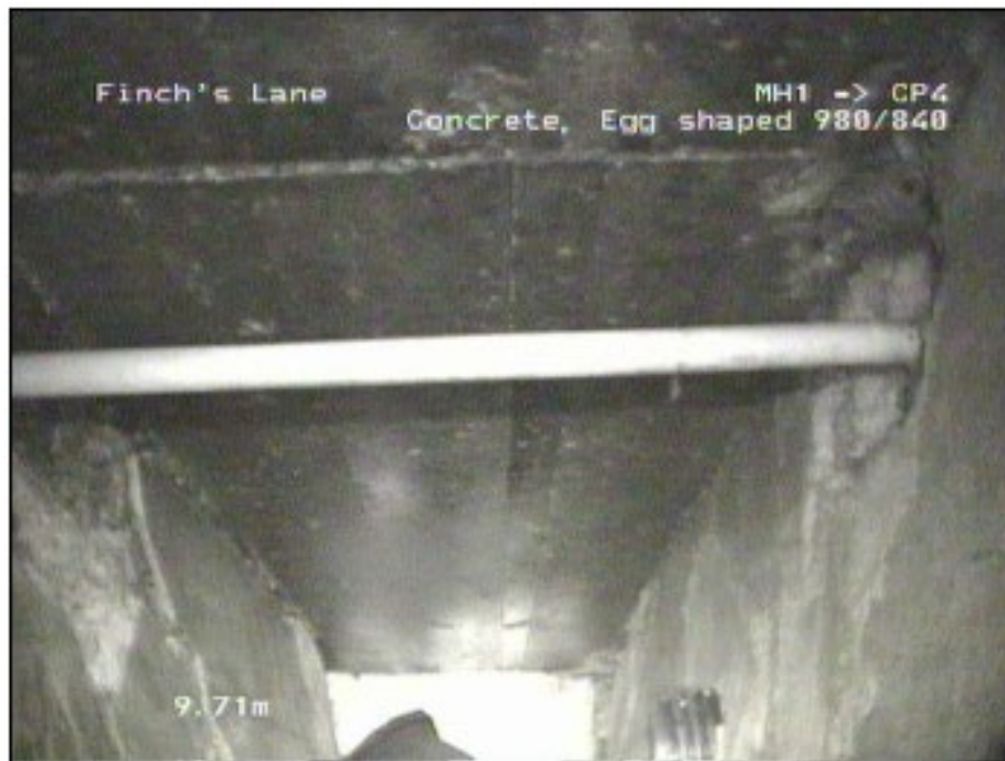
Figure 3.3 – Utility connection
