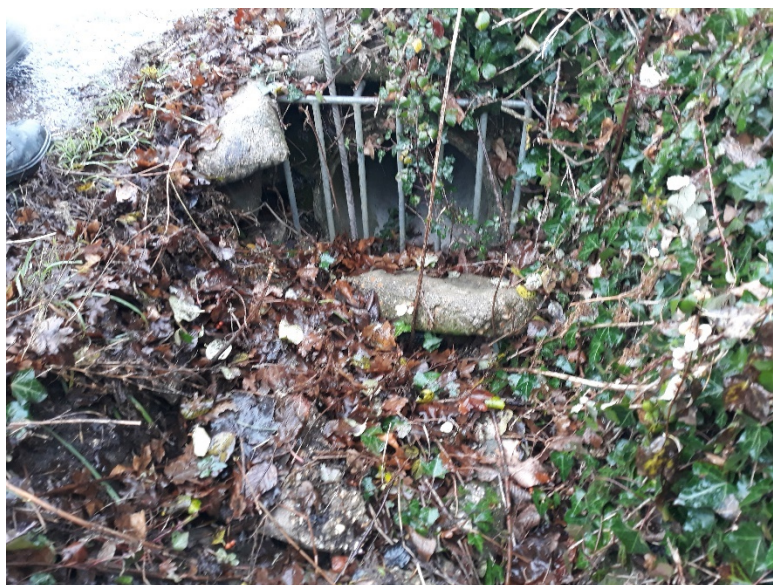
Figure 3.6 – Concrete Sandbag Headwall
