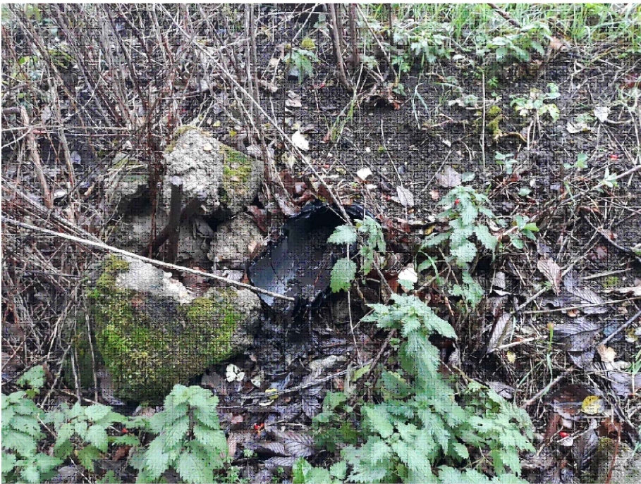
Pipes from road drainage in poor condition and large amount of concrete debris in ditch
